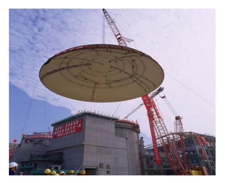
Fig. 5.15. Lifting of dome module (Lingao).
