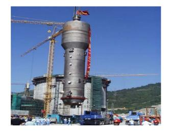
Fig. 5.5. Steam generator installation (Qinshan).
