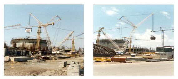
Figs. 5.6. & 5.7. End shield and calandria installation (Tarapur).
