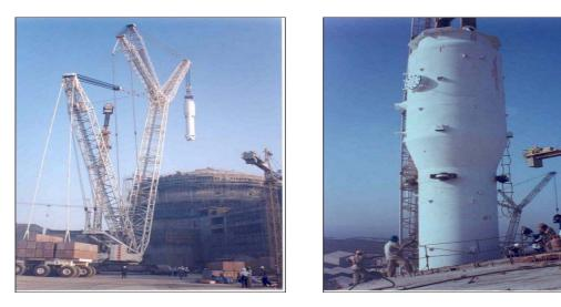
Figs. 5.8. & 5.9. Steam generator installation (Tarapur).
