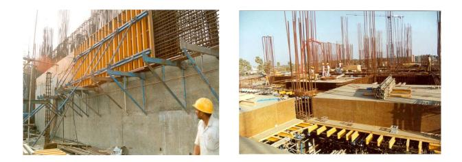
Figs. 5.21. & 5.22. Doka shuttering installation in wall & slab (Tarapur).
