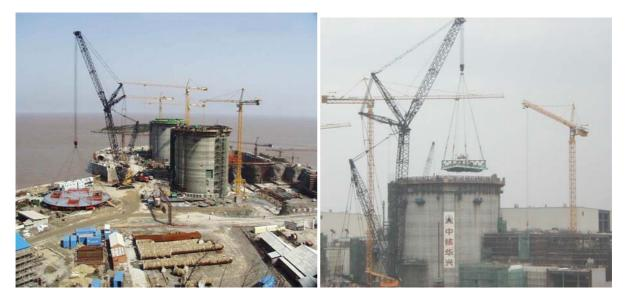
*Figs. 5.3. & 5.4. VHL crane lifting the temporary roof and dousing module (Qinshan).*
