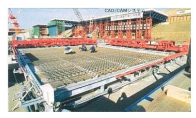
Fig. 5.20. Automatic rebar assembly machine (Kashiwazaki-Kariwa).
