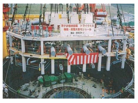
Fig. 5.10. Installation of upper drywell super large scale module (Kashiwazaki-Kariwa).
