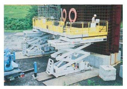
*Fig. 5.19. Automatic elevating scaffolding & horizontal rebar feeding machine (Kashiwazaki-Kariwa).*
